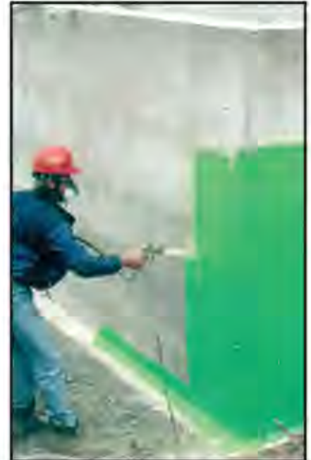
Above: Rub-R-Wall applied with pressure spray.
