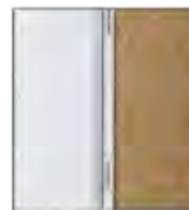
Staple division molding to subwall along resealed edge.
