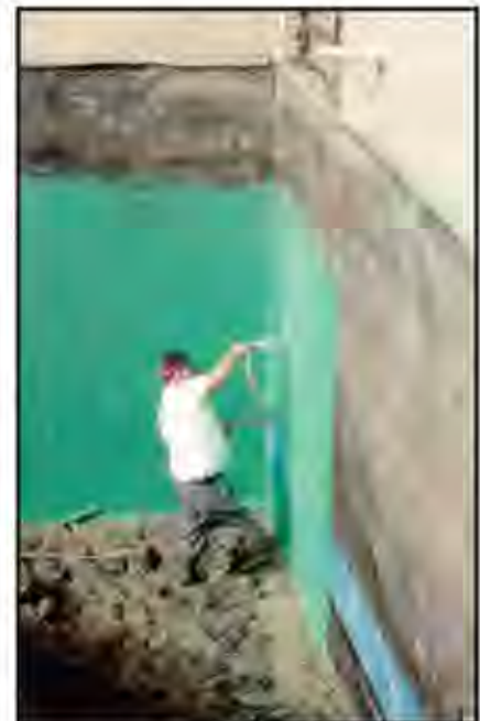
Above: Rub-R-Wall installed in retrofit application.
